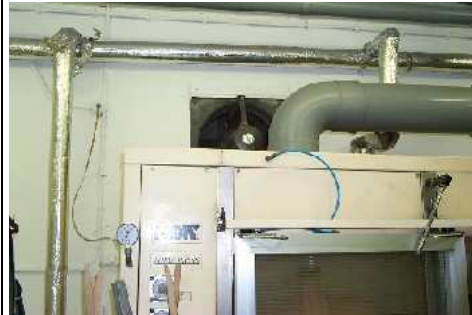
Afzuigventilator in wand
